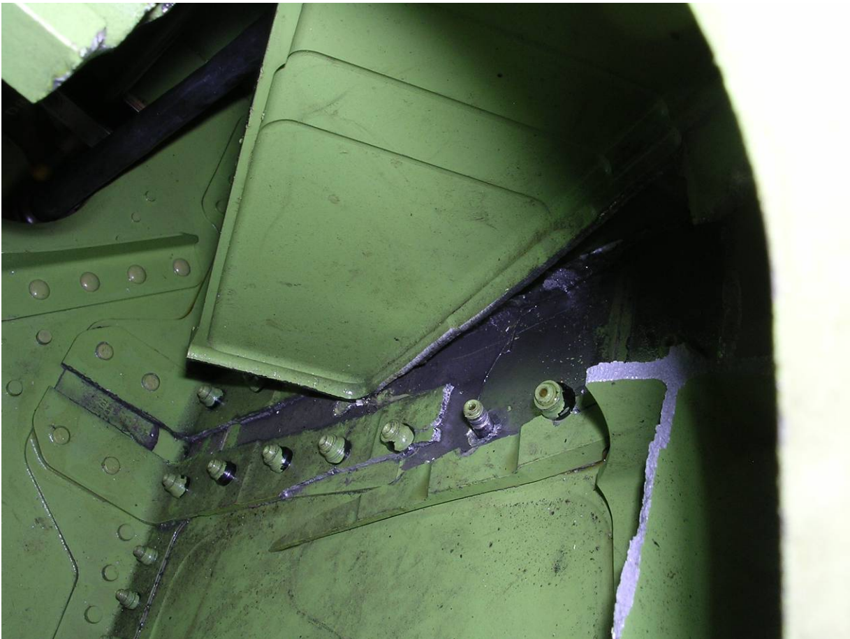
Photo 1: Right wing, support fitting torn out
