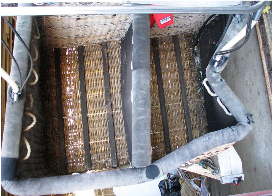
Deformation of the metal railing on one of the compartments
