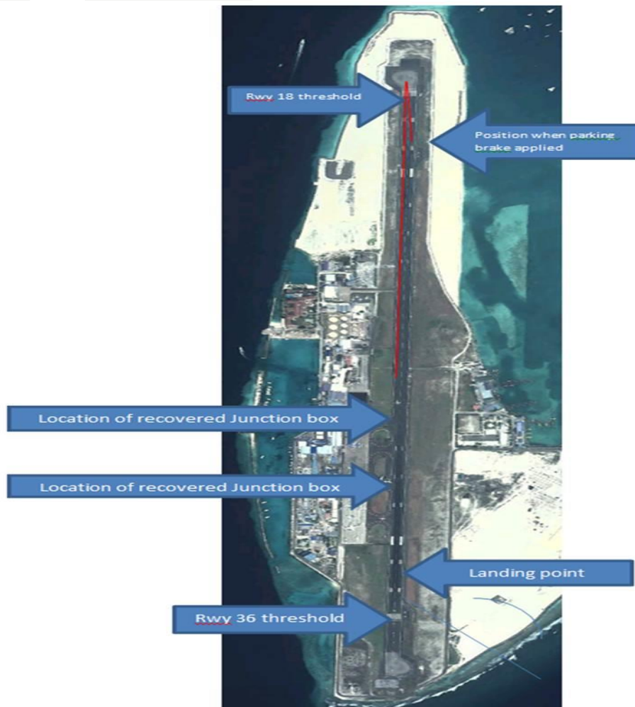
Figure 7. Google Earth image with approximate position of the recovered junction boxes, runway damage and the landing point.
