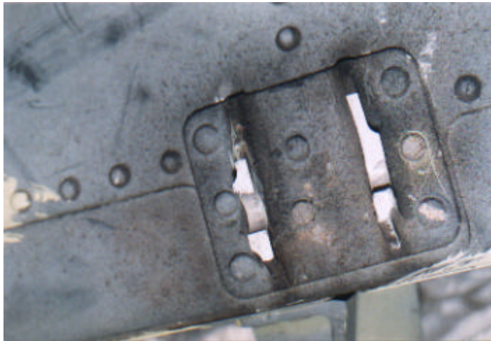
Figure 1B. Broken Fitting on Ventral Door Structure (13 fittings)
