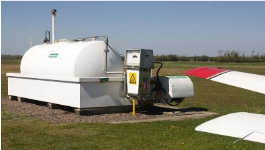
Fig.5. Storage tank installation at Sjöbo/Sövde airfield.
