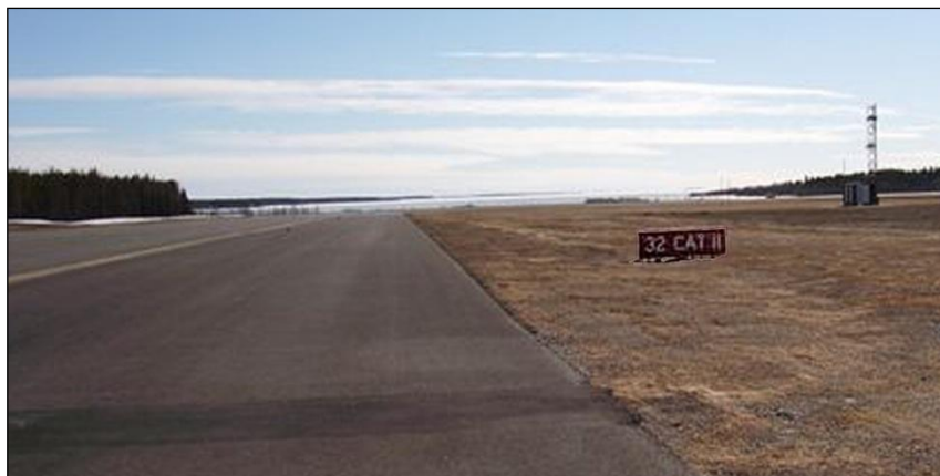
Figure 7. Holding position for runway 32 in CATII conditions
